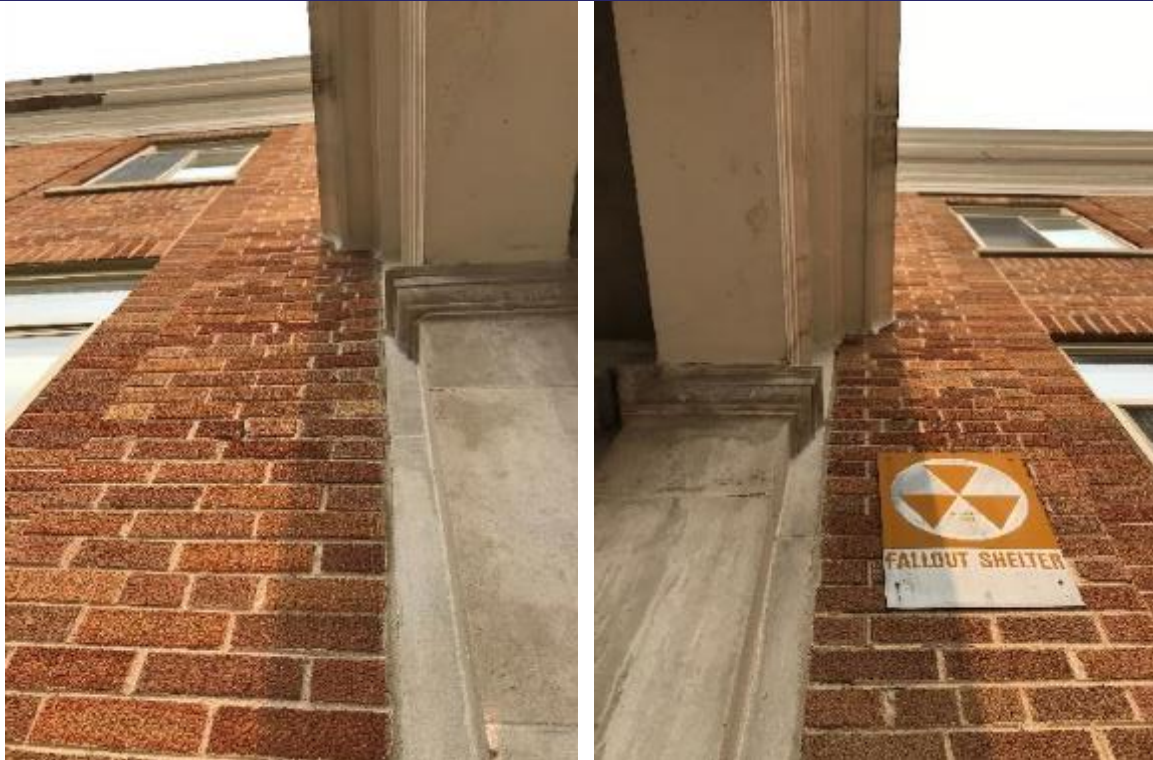
Tuck pointing, brick repair and possible kick out flashing at roof/wall intersection needed.
