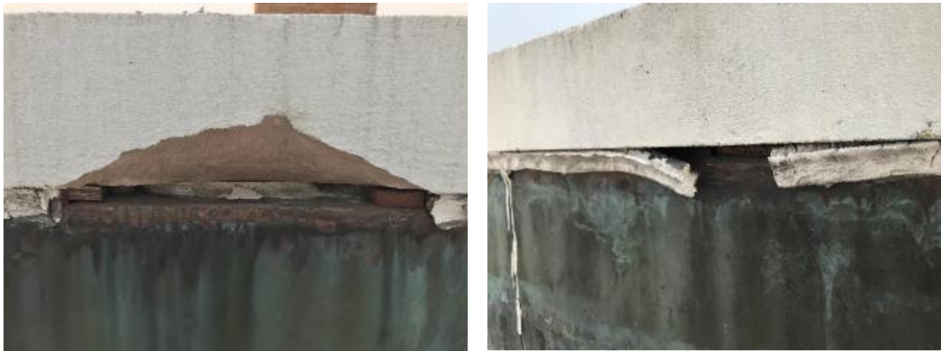
Roof parapet cap sealant and paint repair needed.
