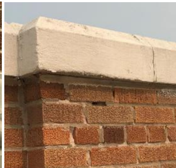
Tuck pointing needed at roof parapet.
