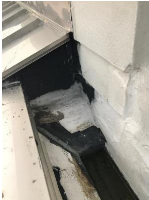
1929/1977 building joint waterproofing repairs needed.
