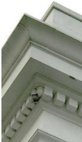
Dentil / paint damage.
