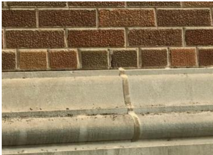
Intersection between brick and decorative stone base where mortar is eroding from water.
