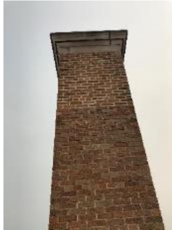
Tuck pointing, cracks and some brick repair needed at chimney.
