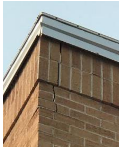
Brick and mortar cracks in veneer likely caused by slight differential movement over time on 1977 building.
