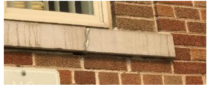
Tuck pointing, brick, decorative stone and paint repair needed.
