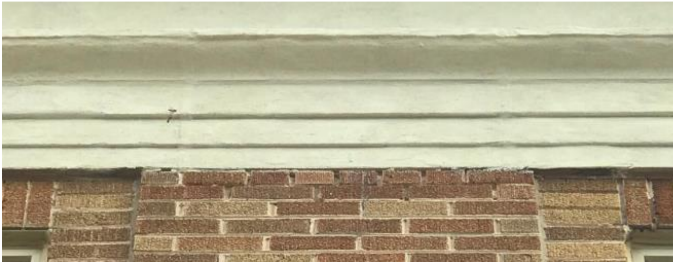
Intersection between brick and decorative stone architrave, mortar and brick has eroded from water.
