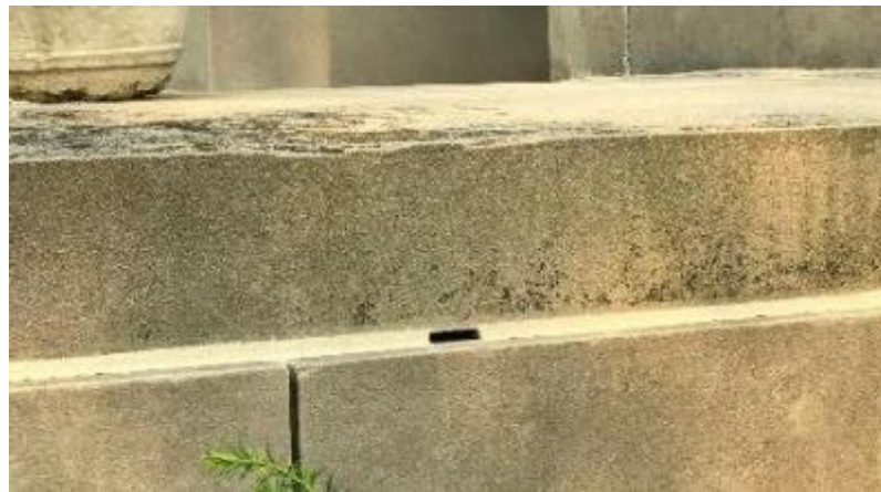
Sealant/caulk repairs needed at portico decorative stone joints.
