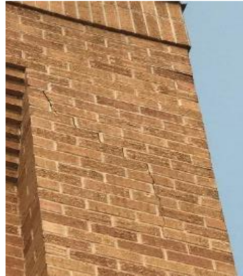
Brick and mortar cracks in veneer likely caused by slight differential movement over time on 1977 building.
