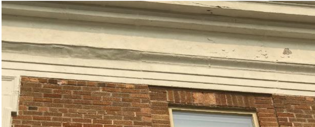
Tuck pointing, brick and paint repair needed.
