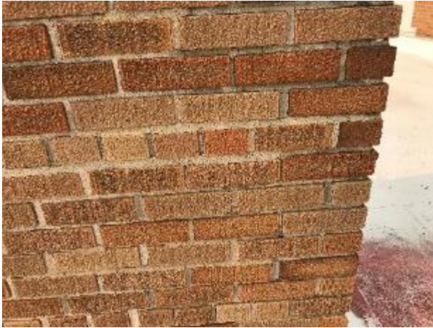
Tuck pointing, cracks and some brick repair needed at chimney.
